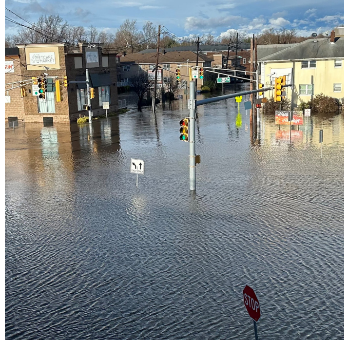
Flooding on Main Street at Route 46 in Lodi Township, Dec. 2023
